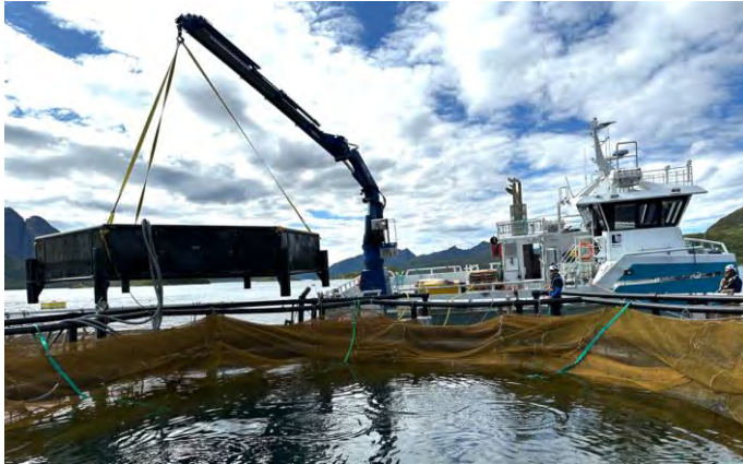
Figure 5d, Docking being lifted in the cage by a farm boat. Figure 5e, Docking mounted with 6x 9T rope shackles.
