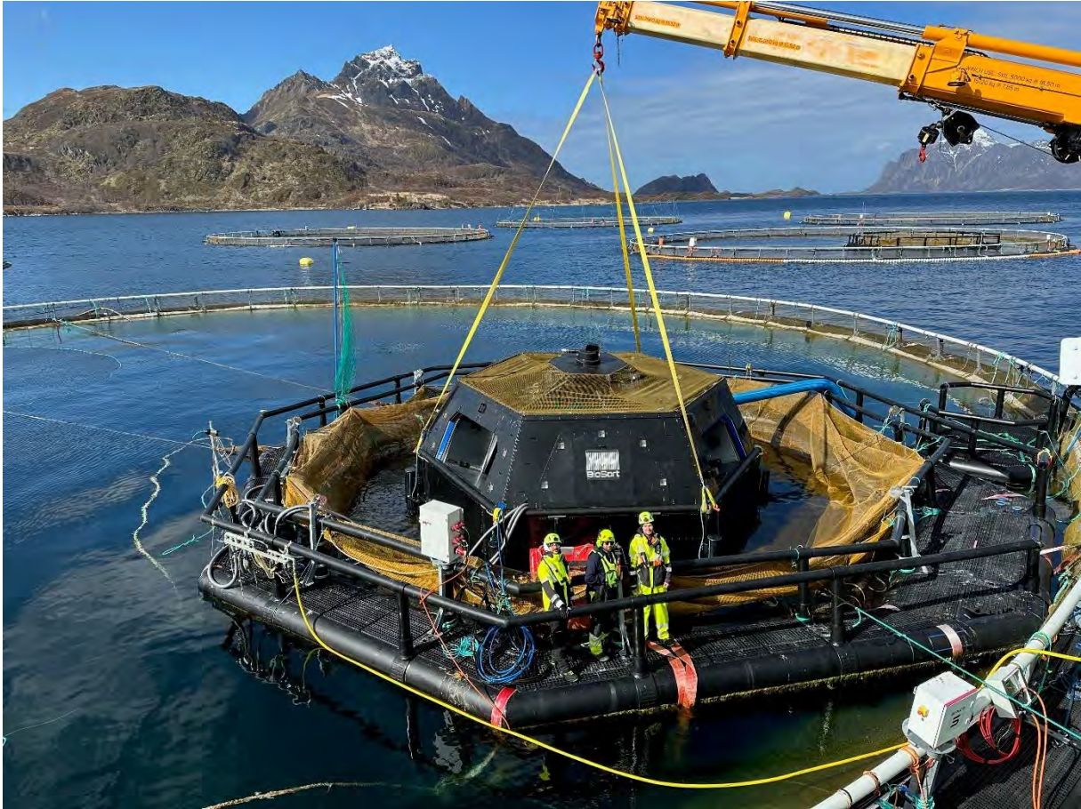
Figure 20: Phase 4 iFarm house installed in commercial cage.
